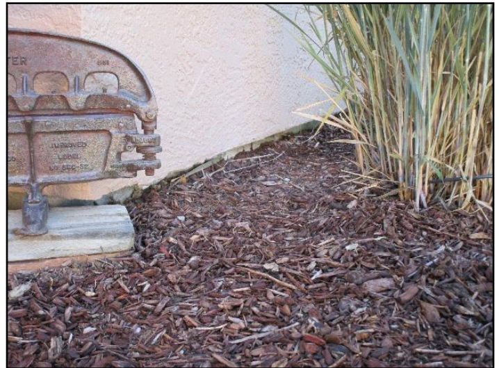
Siding too close to grade
