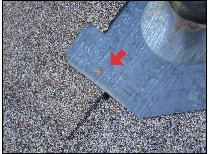
Exposed, missing fasteners
