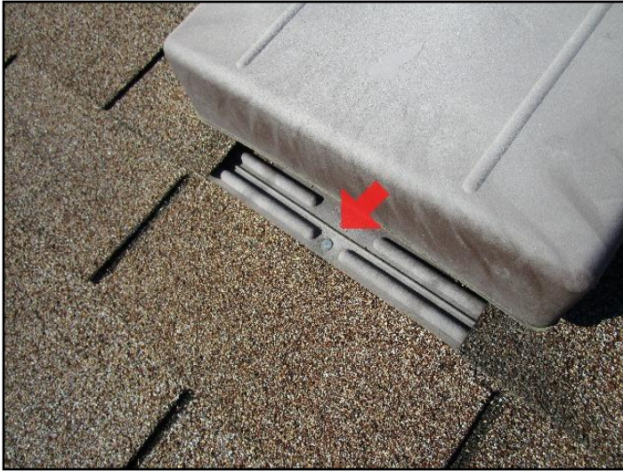
Exposed, missing fasteners
