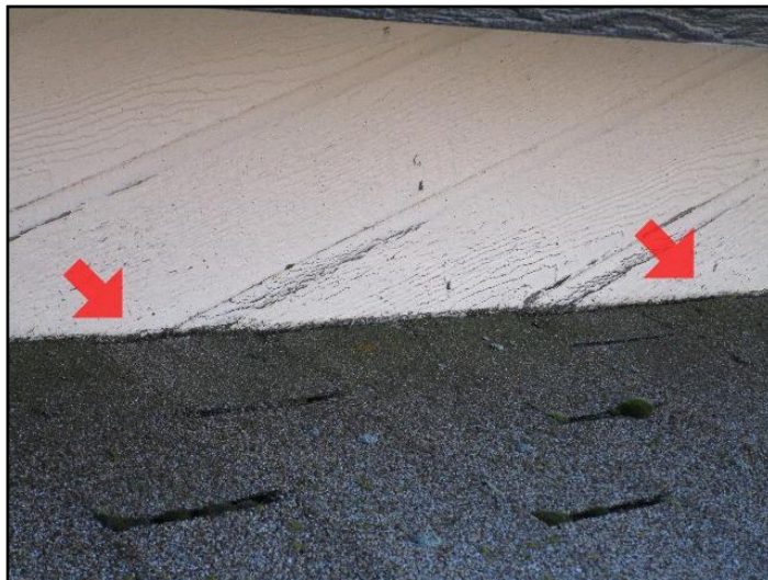
Siding not cut back
