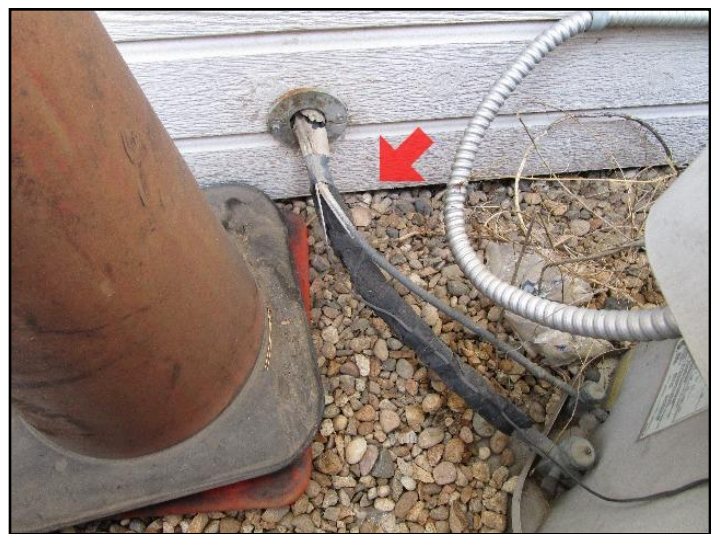
Missing insulation
